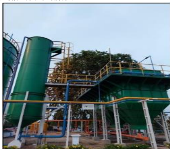
Figure 11. Foam Arrestor and Clarifier Lamellas
